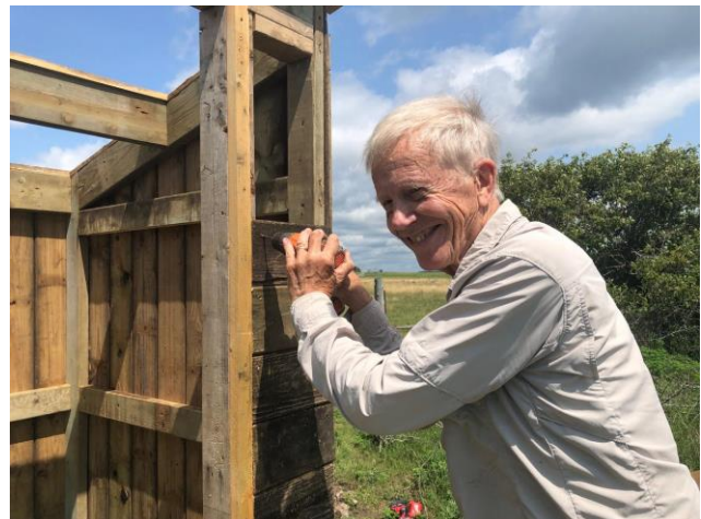
Mike Evans helping put up the outhouse walls.
